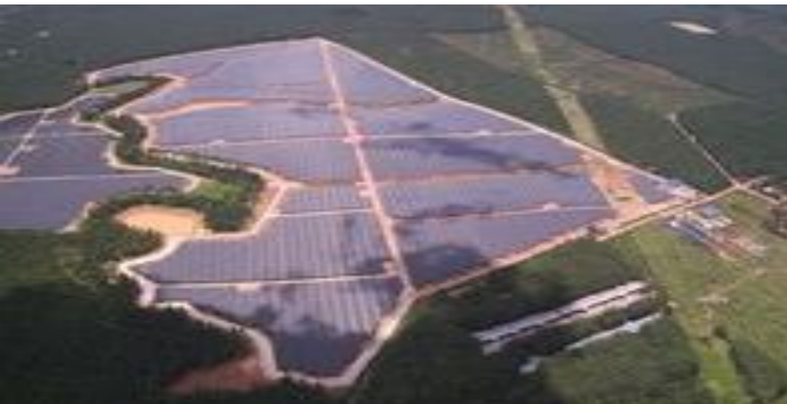
3SP plant Under Construction in Malaysia
