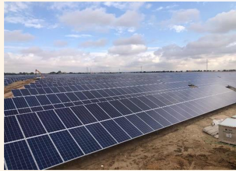
PV Carolinas (Guadalajara) 10 MWp
