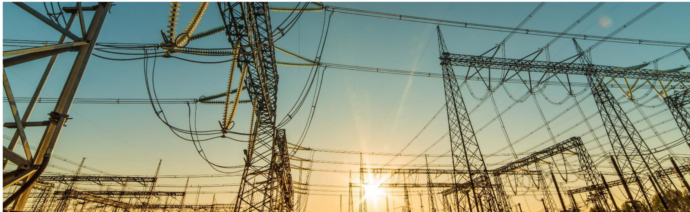
ELECTRIFICATION OF THE ECONOMY AND DIGITALISATION
