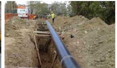
Construction of gas network – Faro, Portugal 1M€
