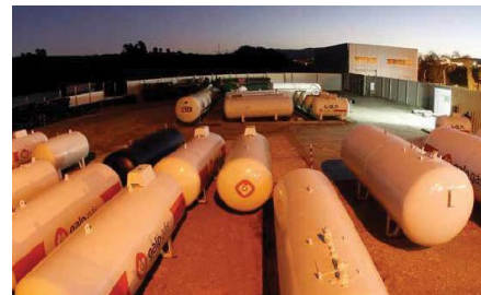
Refurbishment of lpg tanks – Portugal 800K€
