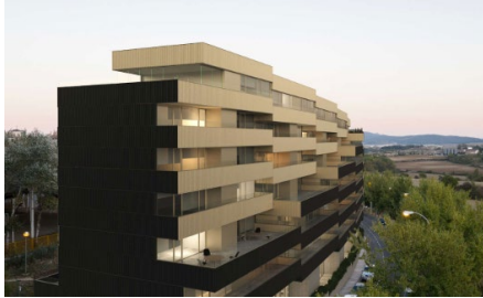
Social housing – Navarre, Spain. 7M€ - In execution
