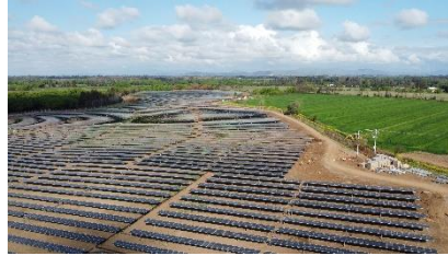
Quinantu (12 MW) Build & Sell - Chile
