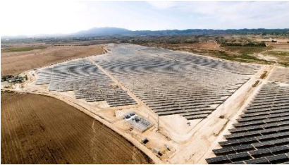
Algibicos (49 MW) Third Party EPC - Spain
