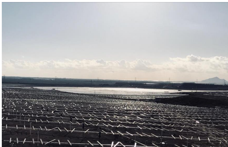
Algibicos plant under construction in Spain
