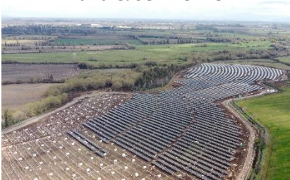
Quinantu (12 MW) Build & Sell - Chile
