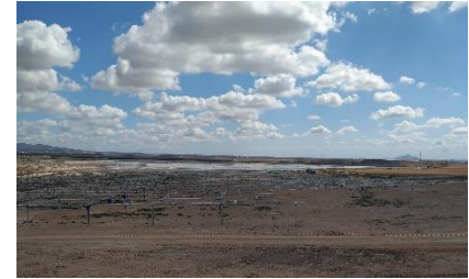
Algibicos (49 MW) Third Party EPC - Spain
