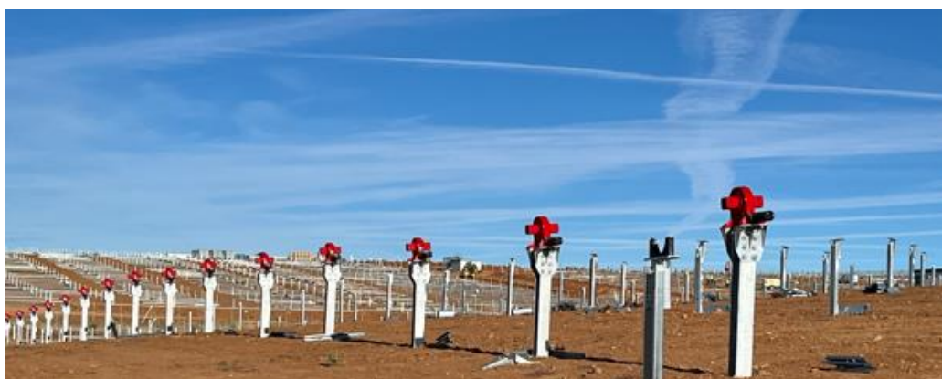
Construction of Cuatro Caminos 1, 2, 3 and 4 projects.
