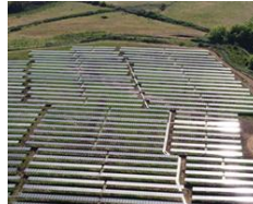
Quinantu 12 MW Build & Sell Chile
