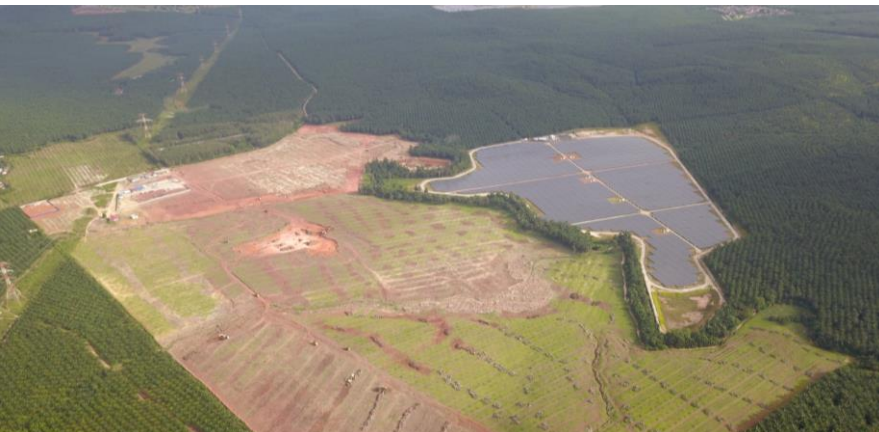
3SP plant Under Construction in Malaysia
