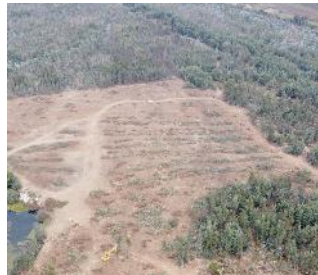
San Antonio* 12 MW Build & Sell Chile
