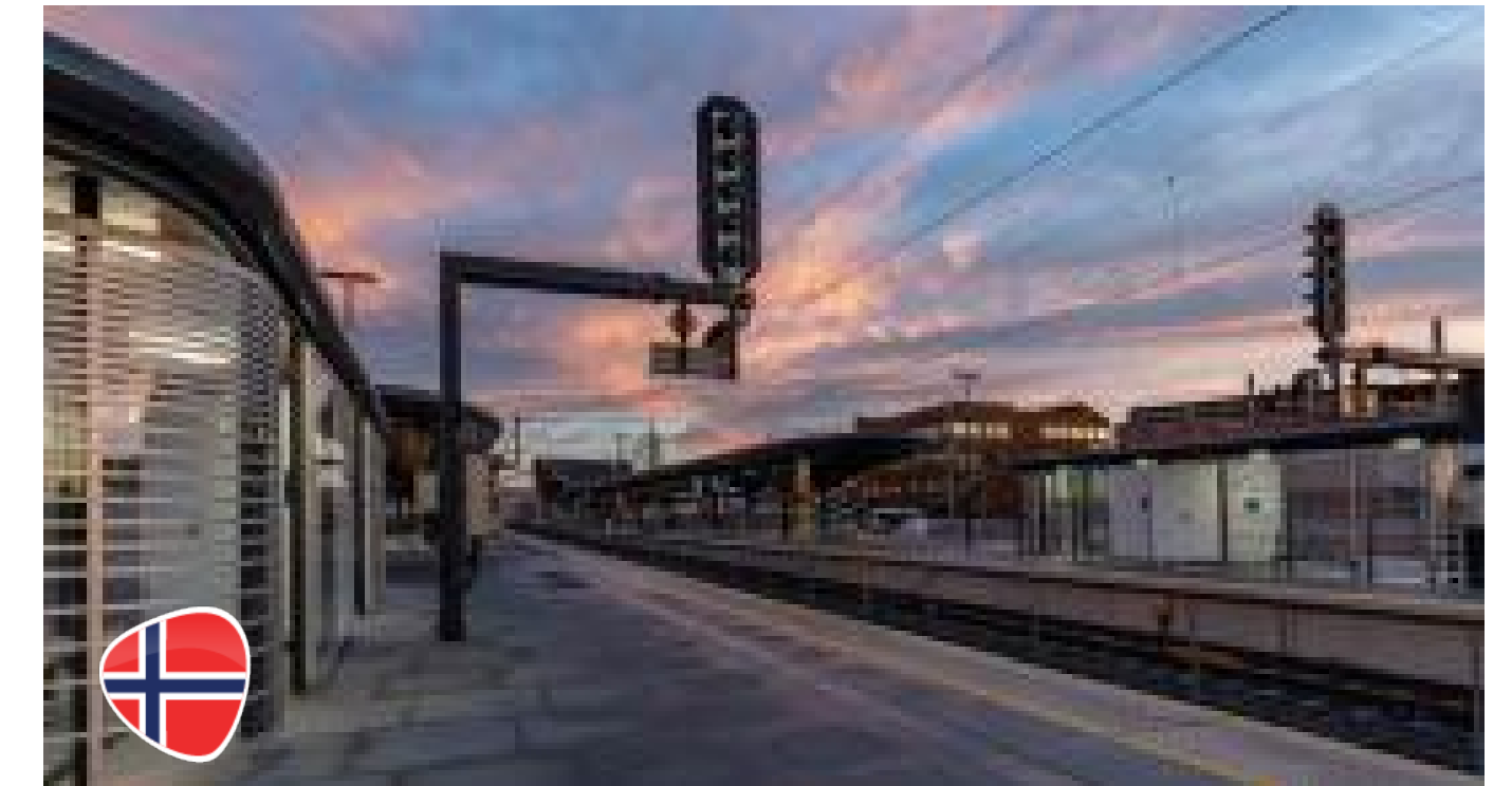
EPC SKI, integrated in the Follo Line high speed line. Project incorporating BIM methodology
