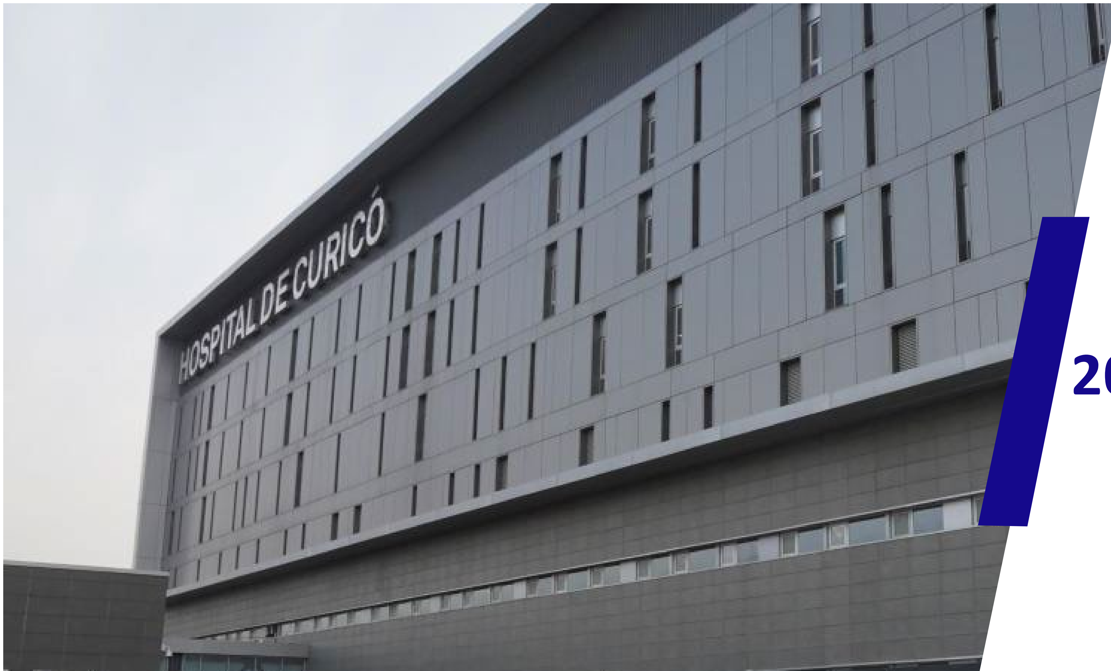
Curicó Hospital. Chile
