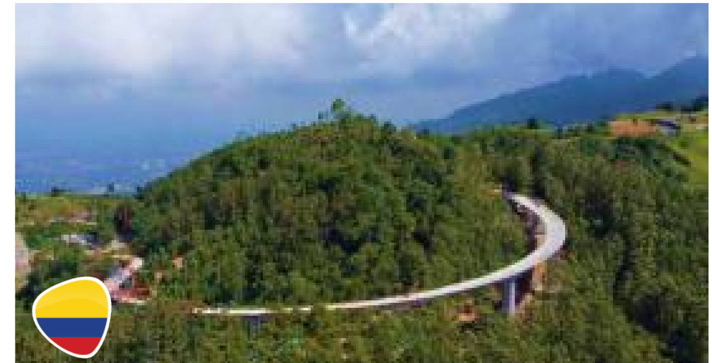
We participated in the construction of the most important road infrastructure in Colombia, the Central Cordillera Crossing
