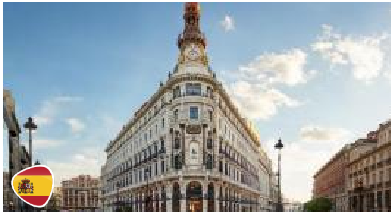
Canalejas. Urban development that promotes a city model aligned with the 2030 Agenda
