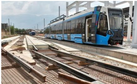
Metropolitan train – Cochabamba, Bolivia 167M€ - In execution
