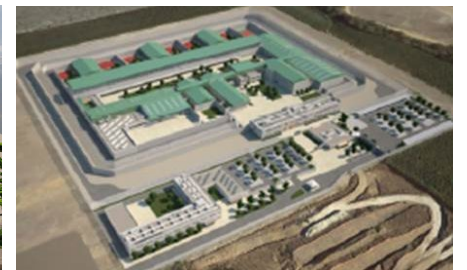
New penitentiary centre – S.S., Spain 39M€ - In execution
