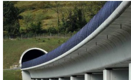
High-speed Pamplona-Zaragoza – Spain 17M€
