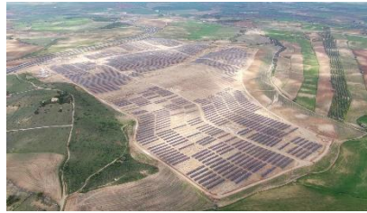
Bargas (50 MW) Third Party EPC - Spain
