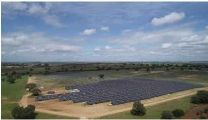
Alvarado (100 MW) Build & Sell - Spain
