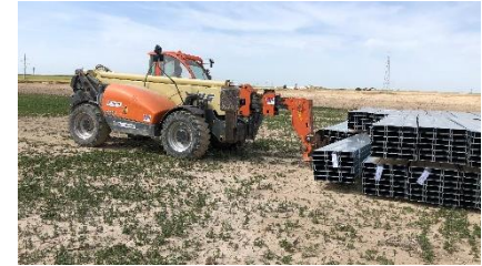
Algibicos (49 MW) Third Party EPC - Spain
