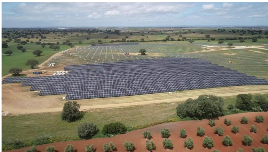
Alvarado plant under construction in southern Spain
