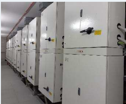
SELF Project in Melilla. Energy storage in second-life batteries.
