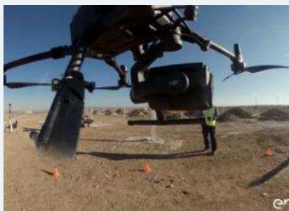
Use of drones to monitor the construction process.
