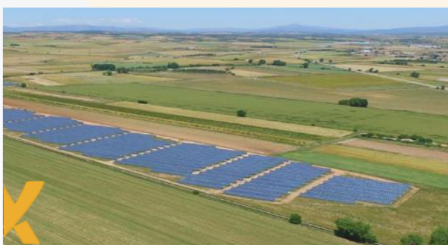
PV Cañamares (Guadalajara) 5 MWp
