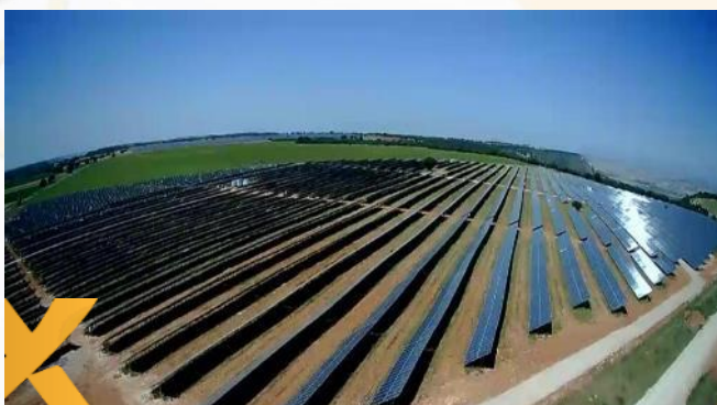
PV Carolinas (Guadalajara) 10 MWp
